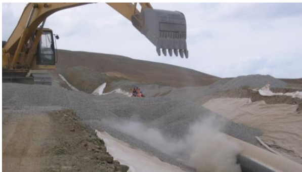
Engineered pipeline fault crossing in construction
