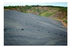
Geomembranes are very low permeability synthetic barriers used to control fluid migration in a human-made system. Geomembranes have been used in forty six (46) different application areas and counting, providing containment in areas such as environmental, geotechnical, hydraulic, transportation, and private development. This lecture will discuss laboratory and field performance of geomembranes related to landfilling of waste.
